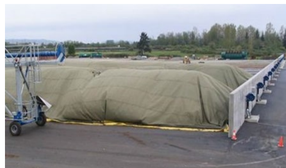
Image: GORE Covered Aerated Static Pile
